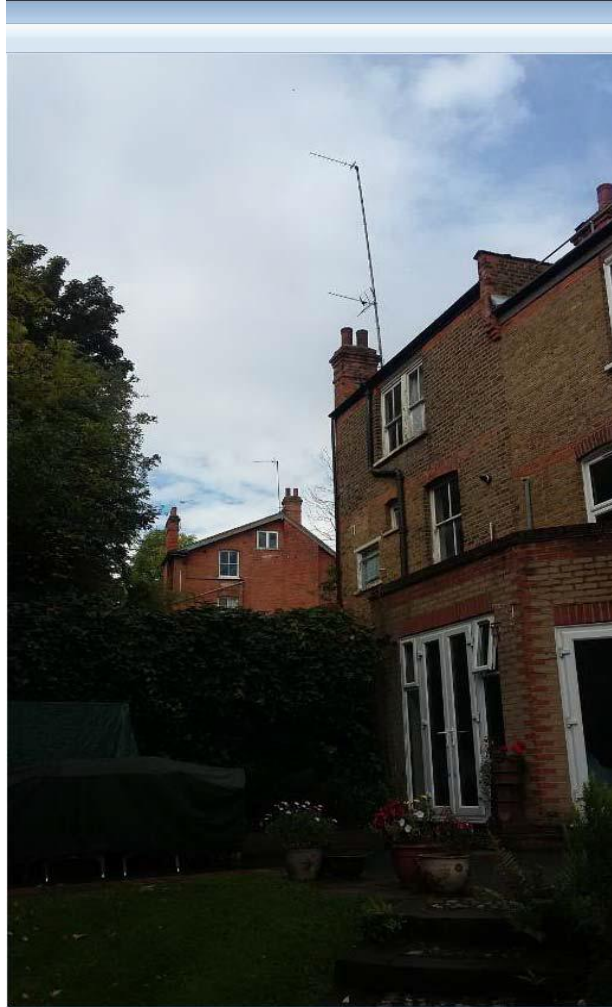
Site photo – rear of the site, (photo taken from neighbouring no. 78 Woodland Gardens)
